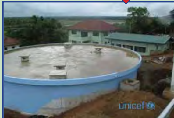
Treated water tank at the new treatment plant
