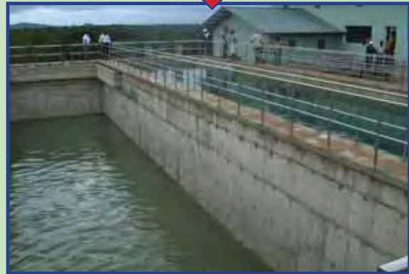
Treated water tank at the new treatment plant
